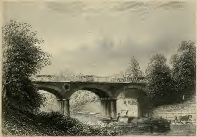
MACCLESFIELD BRIDGE Regent's Park
